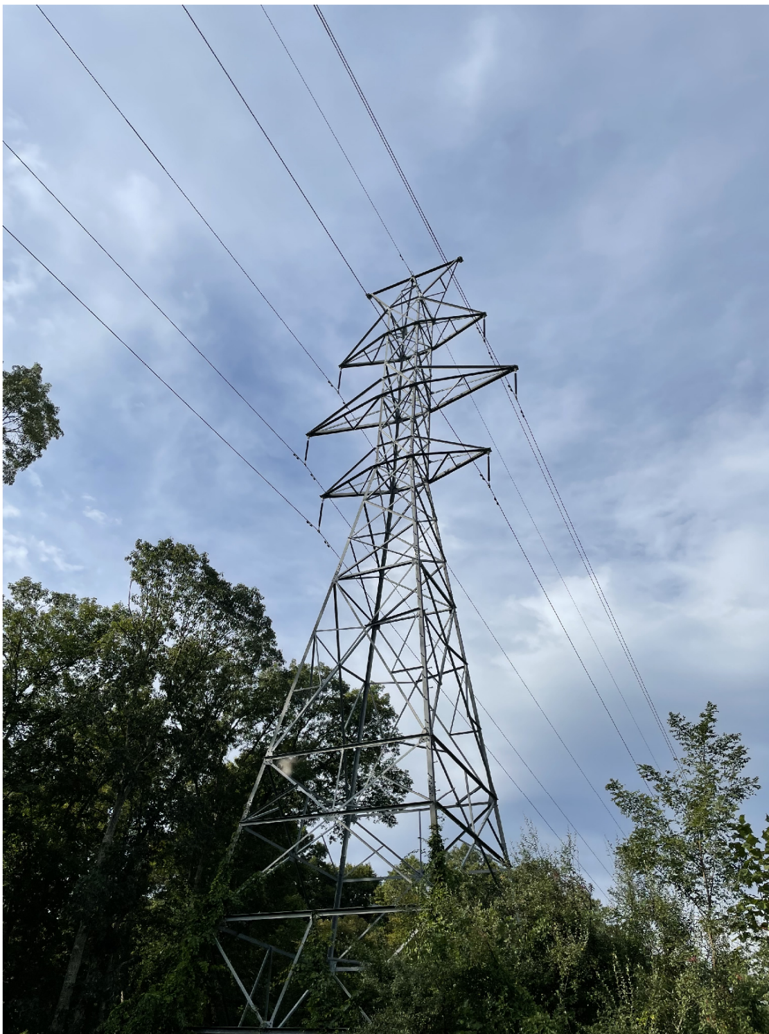
COMPARABLE EXISTING STRUCTURE PHOTOGRAPH
