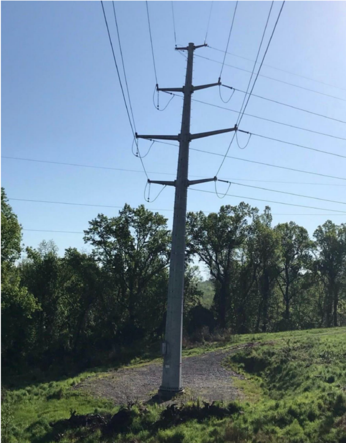
COMPARABLE EXISTING STRUCTURE PHOTOGRAPH
