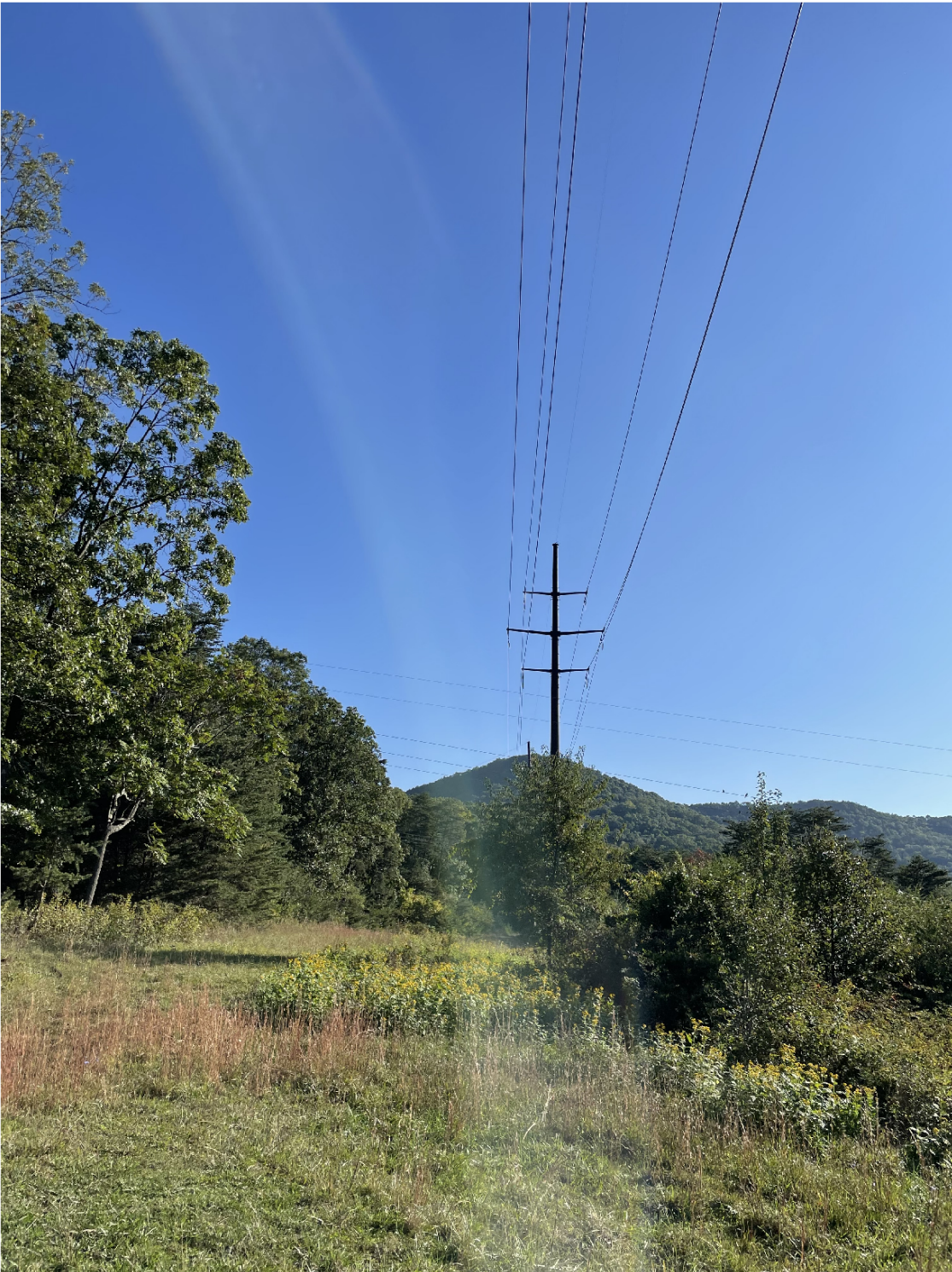
COMPARABLE EXISTING STRUCTURE PHOTOGRAPH
