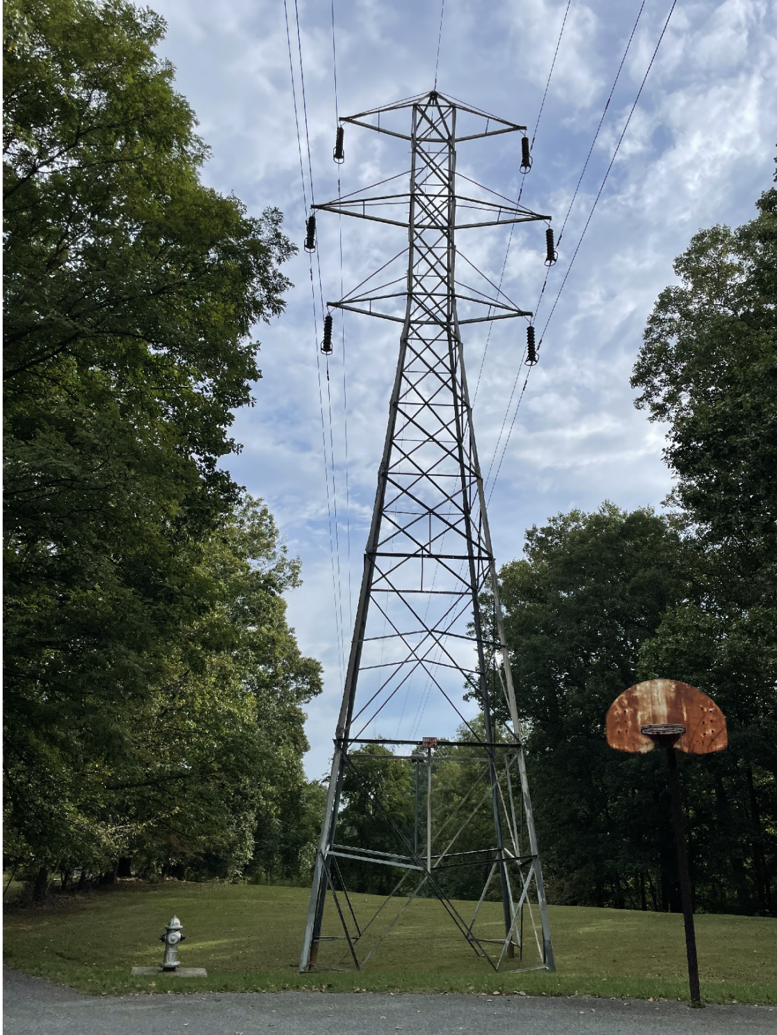
COMPARABLE EXISTING STRUCTURE PHOTOGRAPH
