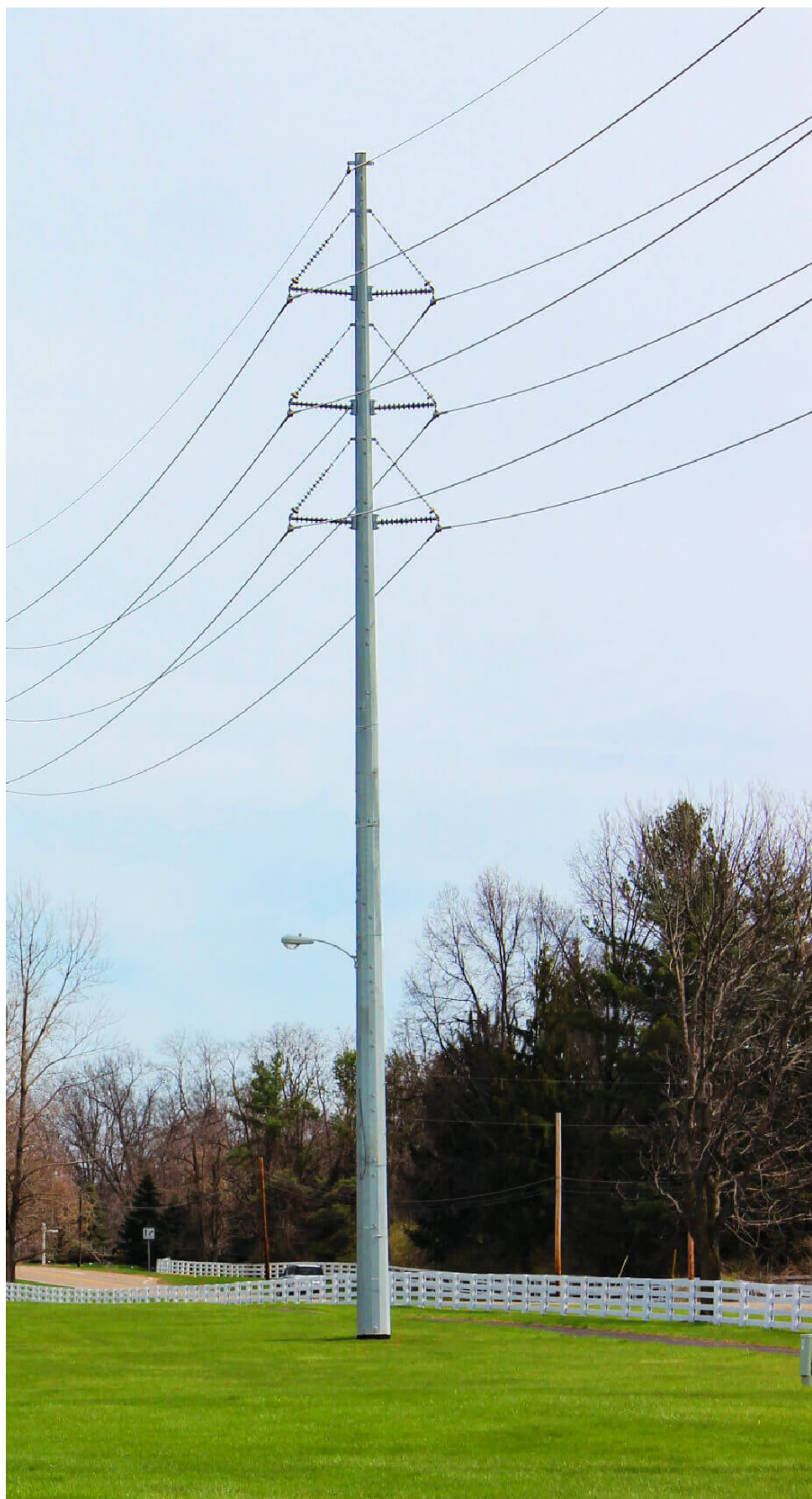
COMPARABLE EXISTING STRUCTURE PHOTOGRAPH
